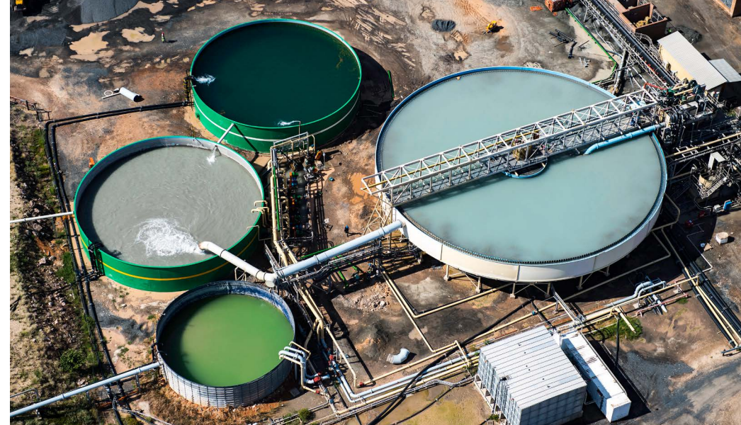
Thickener and processing water storage
