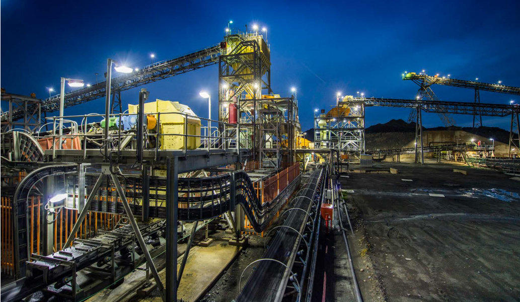
Karowe processing facility and tertiary crusher building
