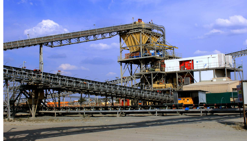
Mega Diamond Recovery (MDR) units
