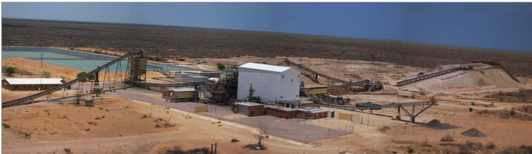
DMS, Recovery, Sorthouse and Tailings Systems
