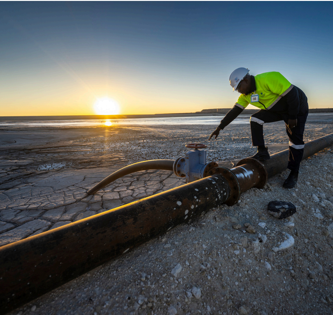
KDM Tailings Storage Facility
