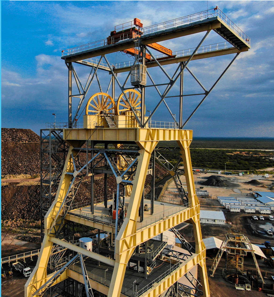
Underground Project at Karowe
