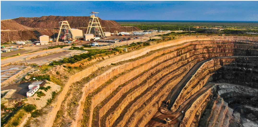
Underground Project view from pit
