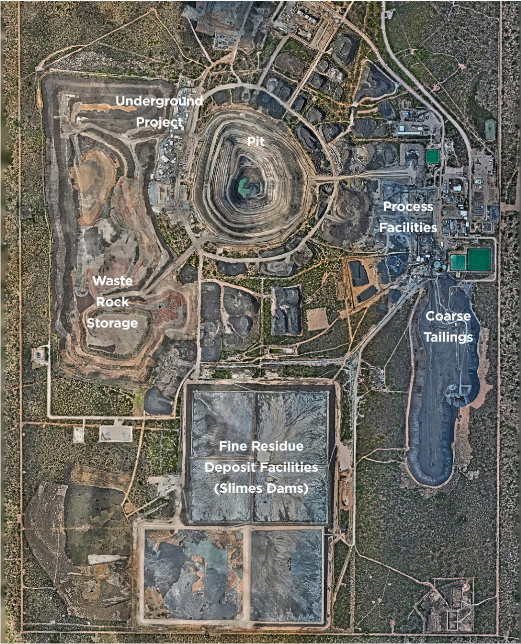
View of KDM Tailings Management Facilities from above
