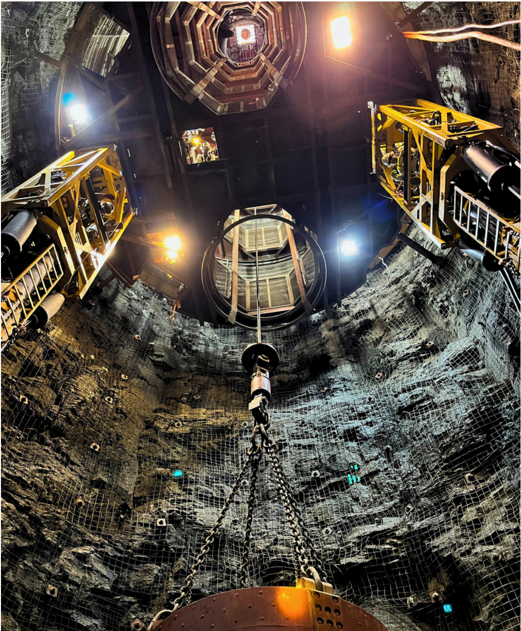
KDM Underground Project
