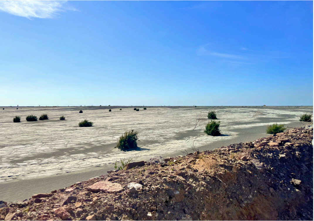
Dewatered tailings at Fine Residue Deposit (FRD) Tailings Facility at Karowe Diamond Mine
