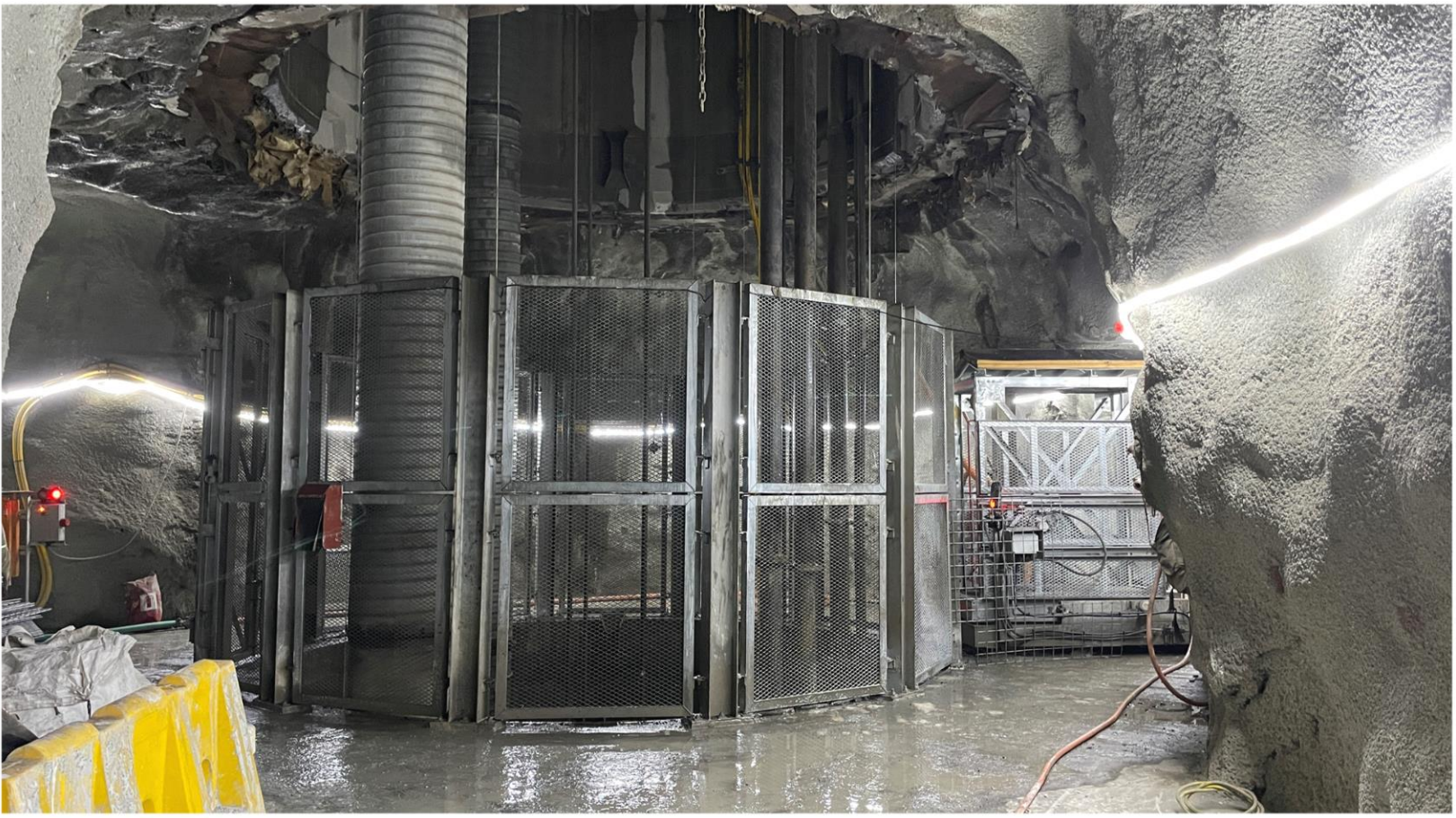
670L Station – Ventilation Shaft
