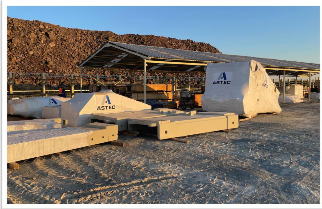
UG Crusher Components delivered to site
