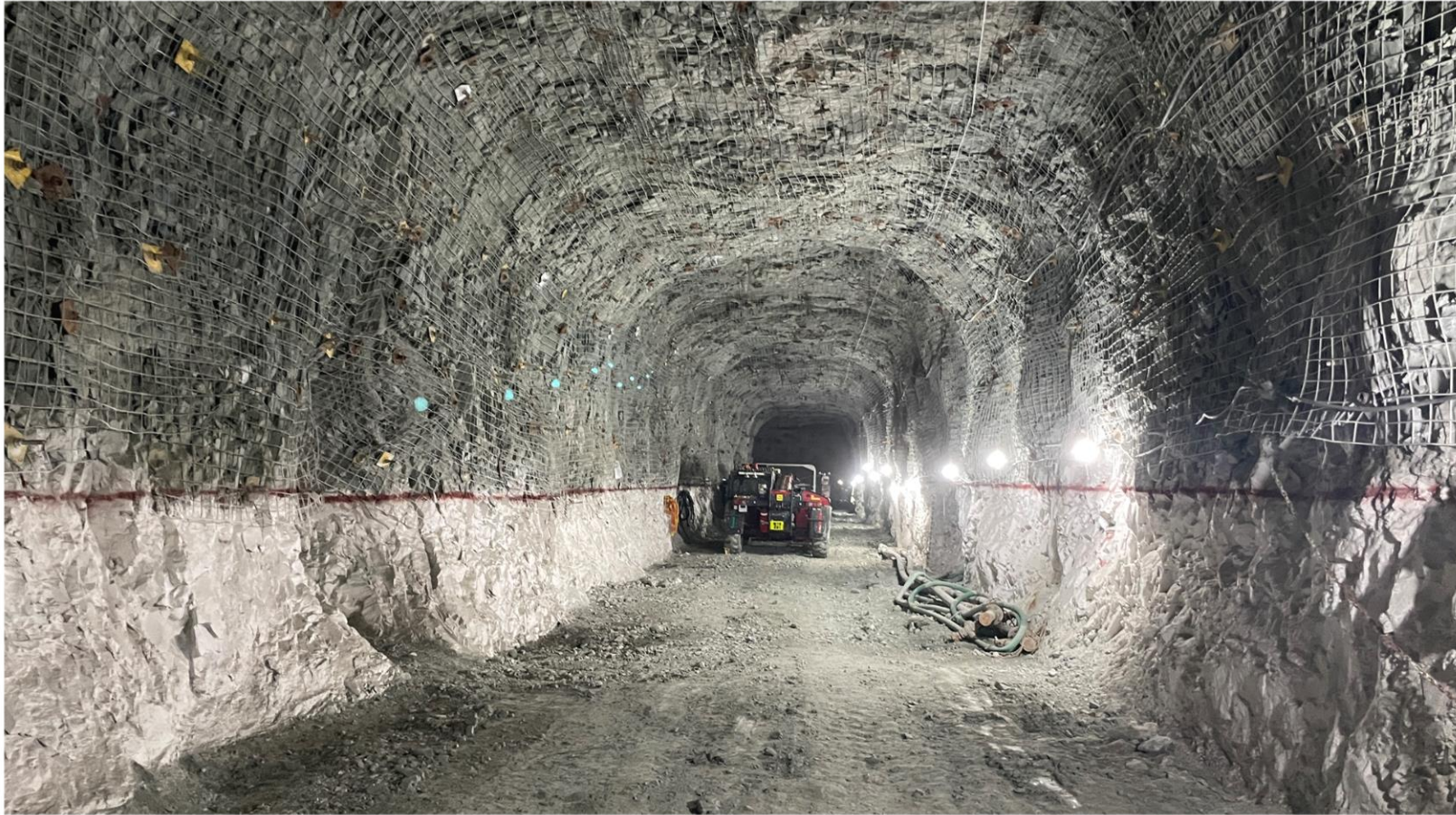
Access 003 – Production shaft to Vent shaft
