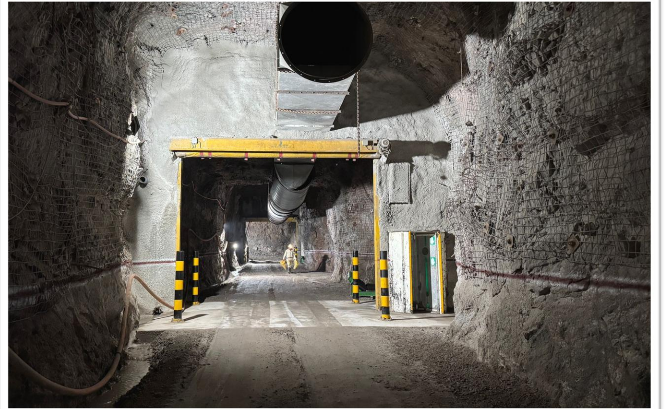
285-Level ventilation shaft doors
