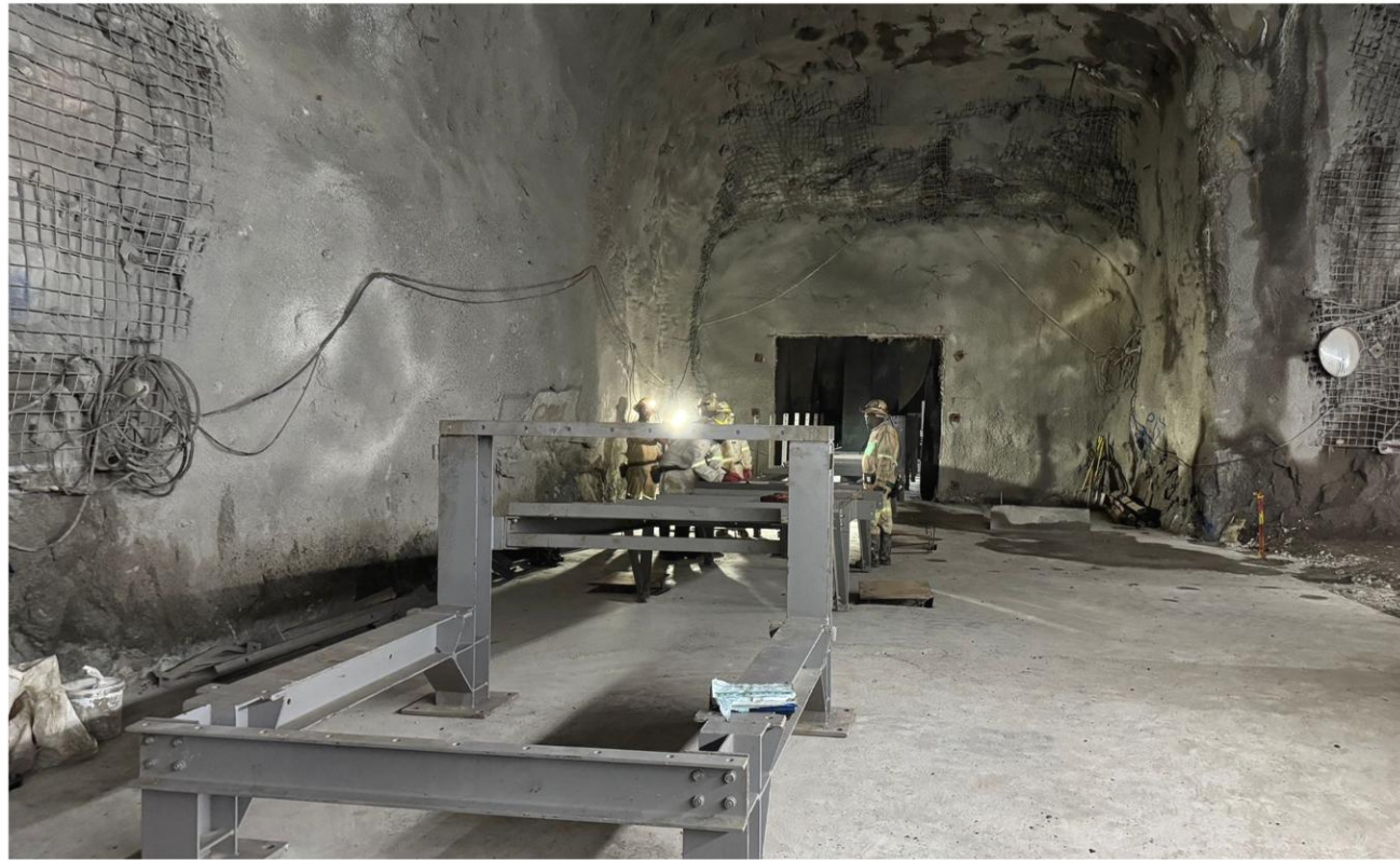
285-Level site loading conveyor structure
