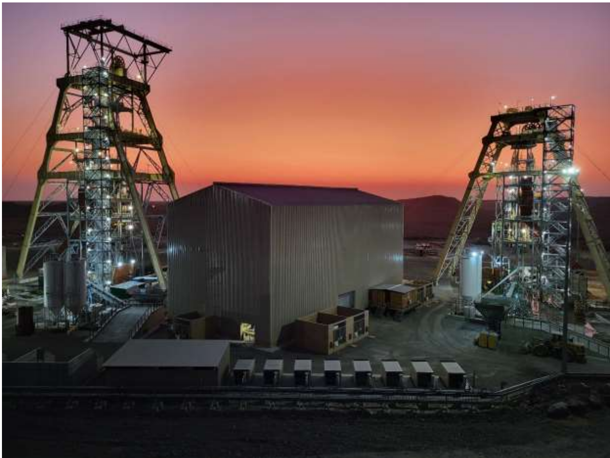
Figure 16-38: Production (left) and Ventilation (right) Shaft Headgear
